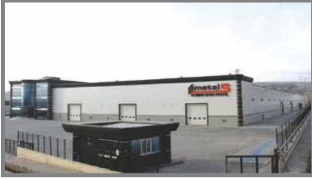
Sonbay Boru Profil Fabrika 1 Sonbay Pipe Profile Factory 1
