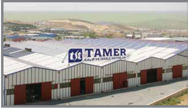
Tamer Kalıp ve İskele Sistemleri Fabrika 1 Tamer Formworks And Scaffolding Systems Factory 1
